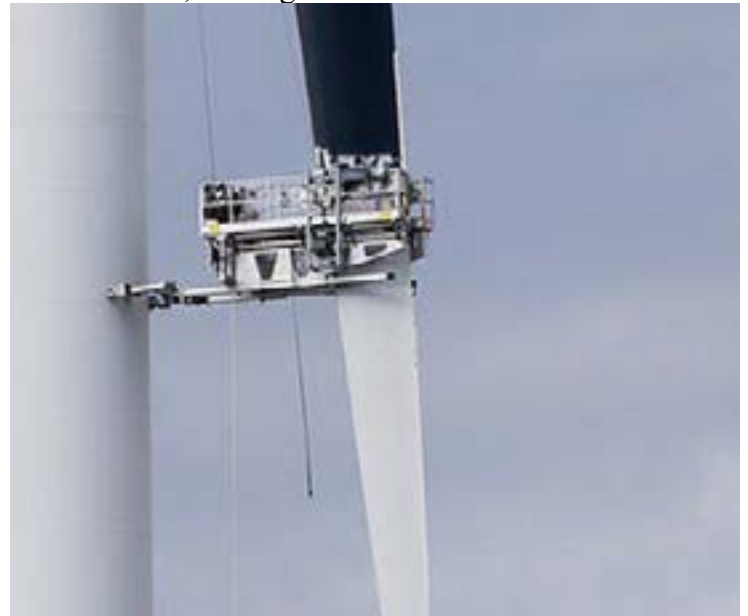
Painting a turbine black (Image: Statkraft)
